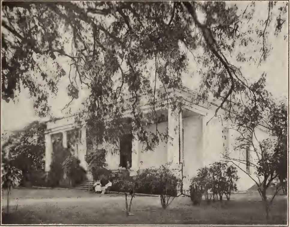
High School Building, Cardenas, Cuba.
